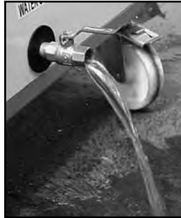
Water Tank Drainage
